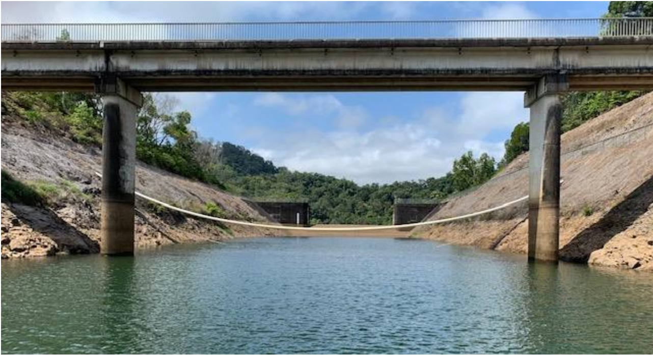
Photo 1- Spillway Net in action at Copperlode Dam.
